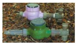
Recycled water is supplied to your home in a separate pipe. Recycled water is supplied through the lilac coloured meter at your property boundary. The drinking water meter is coloured green. From the lilac meter water is distributed through the lilac coloured pipe system.
