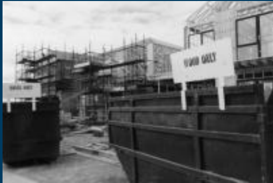
Reducing waste ... more than 90% of construction waste was recycled.
